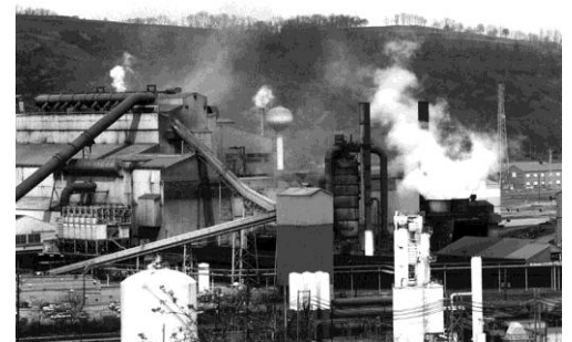
Fairless Works - US Steel Corporation
